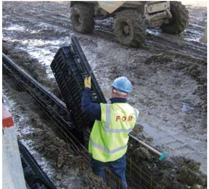
Lightweight elements, installed by one single worker.
